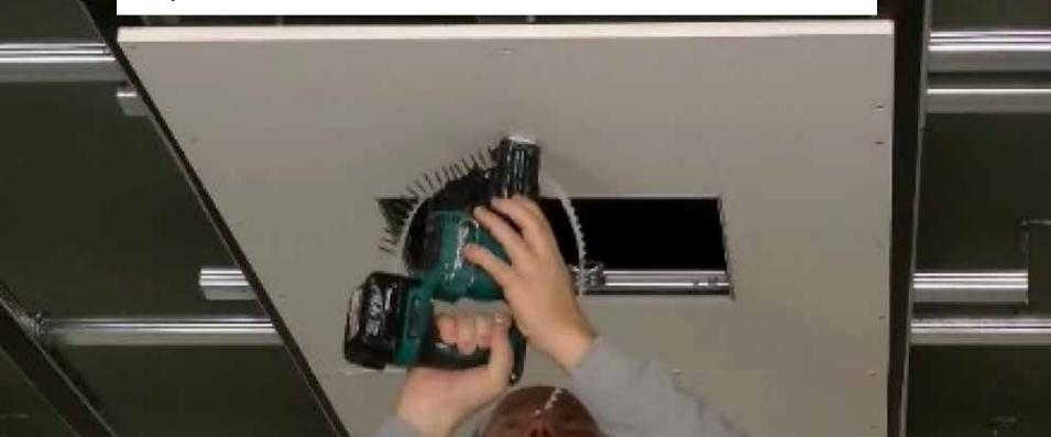
When installing the remaining boards, apply **StarSilent Fix** to all **adhesive edges**. In order to avoid **cross joints**, always install the boards with an offset of at least 400 mm.
