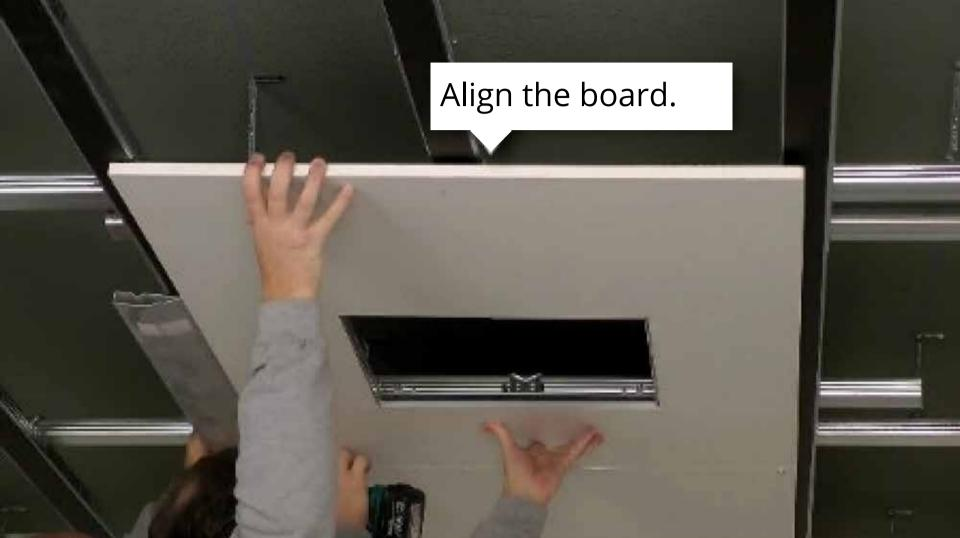
Screw the board to each **fine grid profile**. Screw spacing approx. 200 mm, spacing from edge of board approx. 20 mm.
