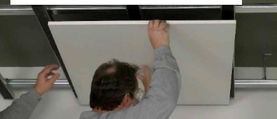
Screw the board to each **fine grid profile**. Screw spacing approx. 200 mm, spacing from edge of board aprox. 20 mm.
