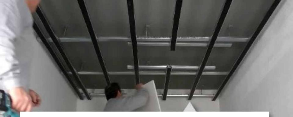
We recommend installing the first board starting from the **2nd fine grid profile** from the wall.
