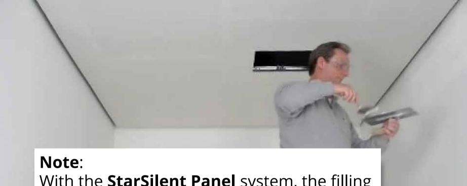
With the **StarSilent Panel** system, the filling of the joints as well as the subsequent work steps have to be repeated until optimum evenness has been achieved (usually twice).
