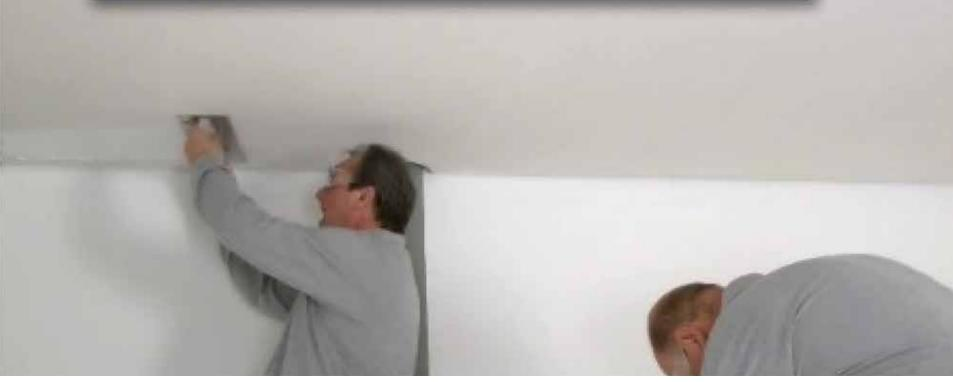
It is important to apply a sufficient amount of material for the subsequent **toothing**.
