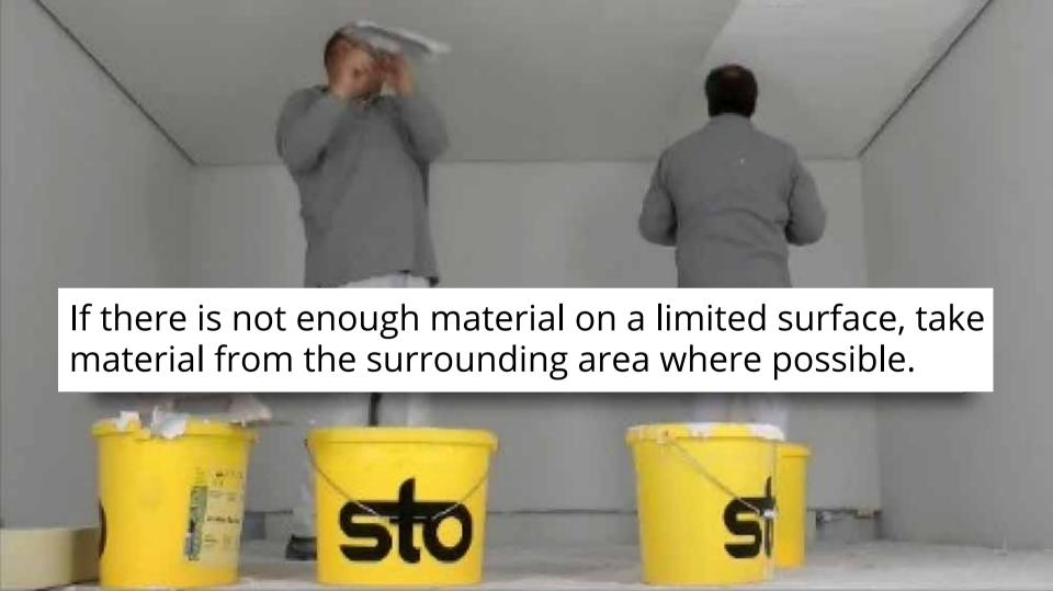
Level the area **along the edges** with the **plastic trowel** after approx. 15-45 minutes (noticeable when the surface becomes matt).
