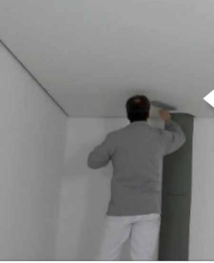
The **plastic trowel** must be continously moistened by means of a **sponge** to remove the emerging **lubricating film** on the tool.
