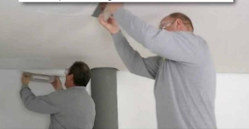
It is important to apply a sufficient amount of material for the subsequent **toothing**.
