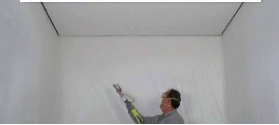
**3 spraying cycles** are usually sufficient. Additional spray layers may be required, depending on the color shade.
